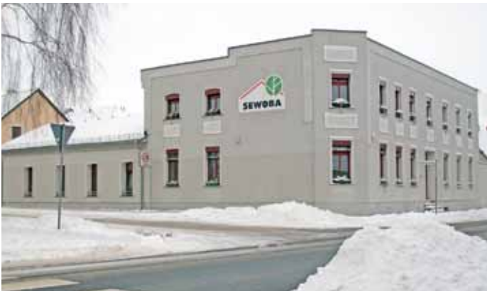
SEWOBA, Küstriner Straße 46 in Seelow
